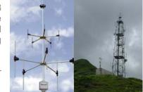
This configuration may be completed by monitoring antennas (omnidirectional or directional) for horizontally polarized transmissions.
